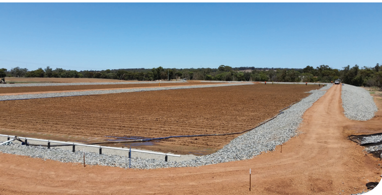
2ha wetland under construction – pre planting
