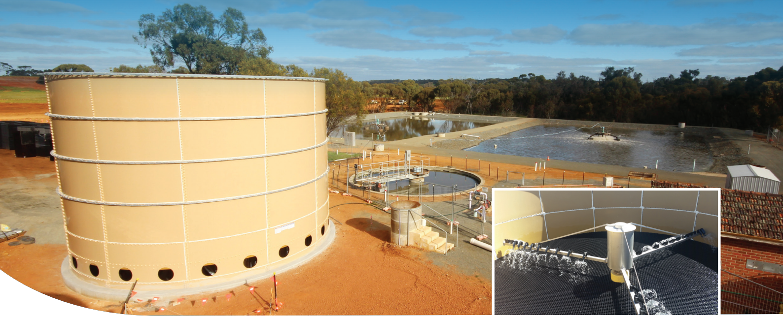
Narrogin WWTP – New Plastic Media Trickling Filter
